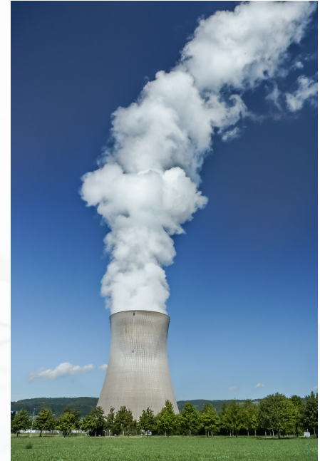
Industrial excess heat is a resource that often goes up in smoke.
